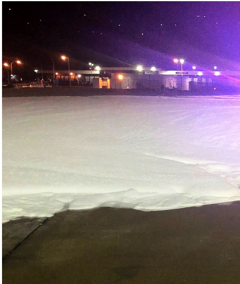
Aftermath of an unwanted foam system discharge. Photo by Author
